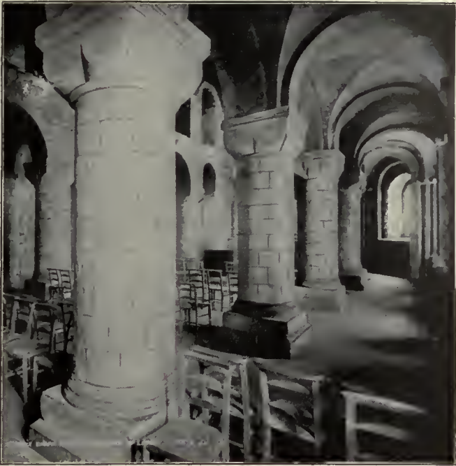
Photo, Valentine & Sons. FIG. 13.—INTERSECTING GROINED VAULTING. Early example. St John's Chapel, Tower of London.
